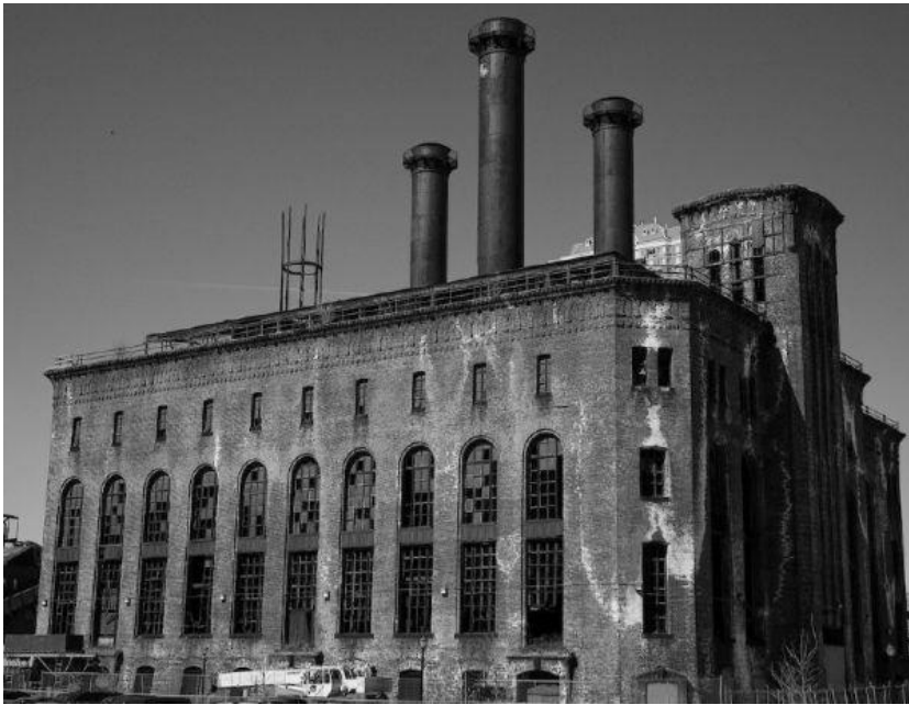
Figure 4 https://i.pinimg.com/originals/dc/da/17/dcda171758eae3ffc268279c98493ccf.jpg : Decaying factory. Source -
